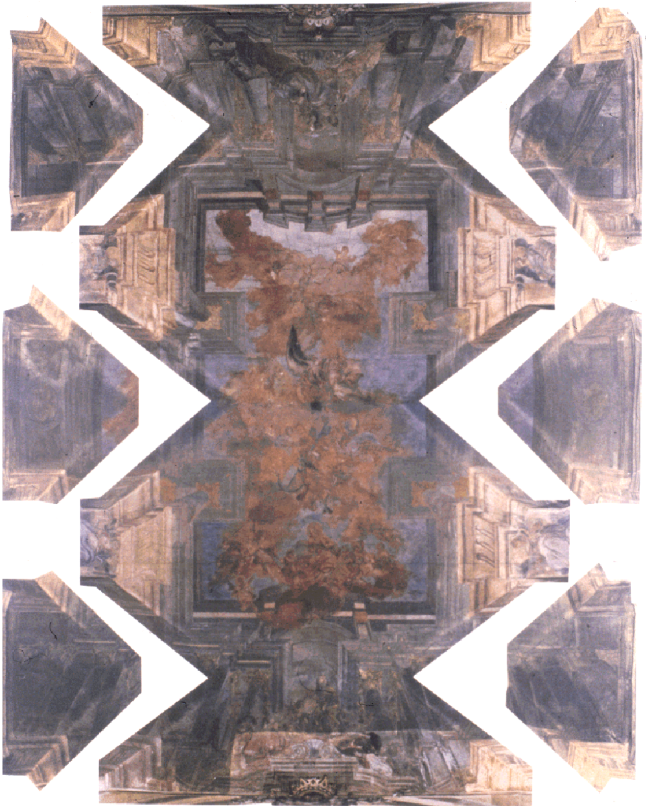
Fig.4. Development of XVIII century frescos from cylindrical vault of Pijar's church in Cracow (Poland) Reproduction of the colour photomosaic (original scale 1:20)
