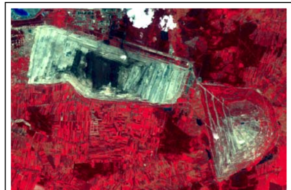
Figure 1. The Belchatow Mining Energy Complex: a) open pit mine, b) dump body and c) power plant
