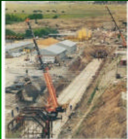
Cut and cover section of Delivery Tunnel North
