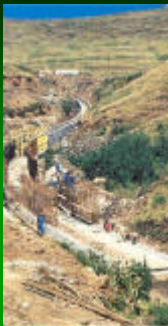
Cut and cover section of Delivery Tunnel North
