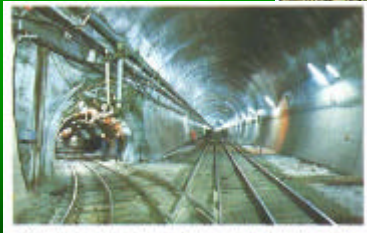
View of main tunnel completed section, showing gallery connect to service tunnel on left side.
