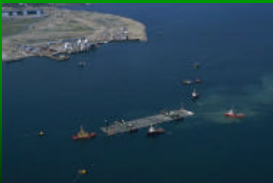
Transport segmentu tunelu
