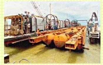
Tunnel elements are constructed in the dry, for example in a casting basin, a fabrication yard, on a shiplift platform or in a factory unit.
