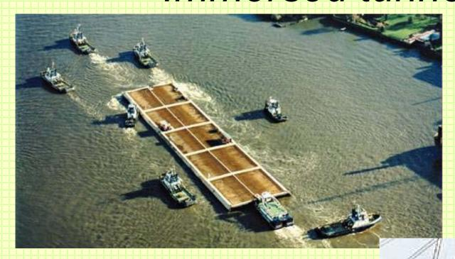
Each tunnel element is transported to the tunnel site - usually floating, occasionally on a barge, or assisted by cranes.
