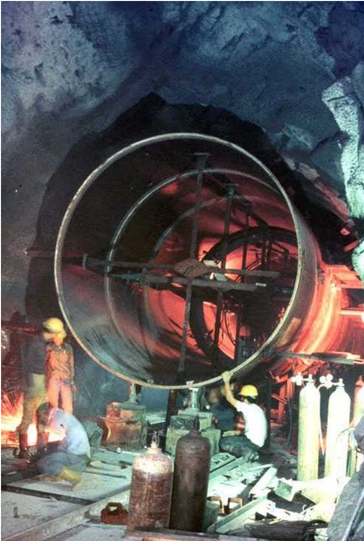
Figure 1.9: Installation of steel lining in a pressure tunnel in a hydroelectric project.
