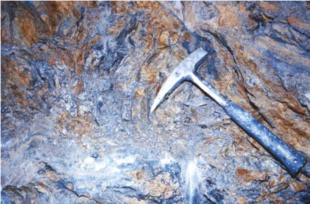
Figure 11.28: Appearance of the very poor quality Athenian Schist at the face of the side heading illustrated in Figure 11.27.
