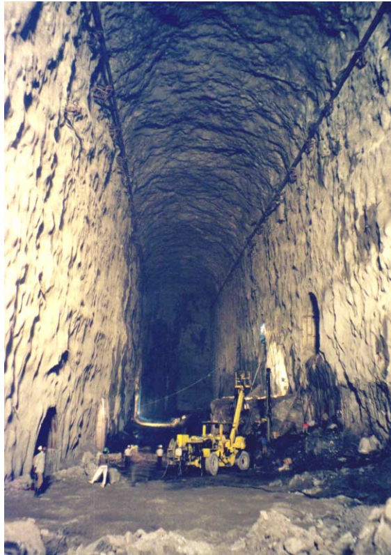
Figure 11.22: Partially completed 20 m span, 42.5 m high underground powerhouse cavern of the Nathpa Jhakri Hydroelectric Project in Himachel Pradesh, India. The cavern is approximately 300 m below the surface.
