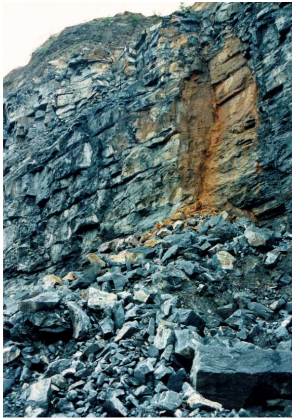
Figure 11.30: Structurally controlled failure in the face of a steep bench in a heavily jointed rock mass.
