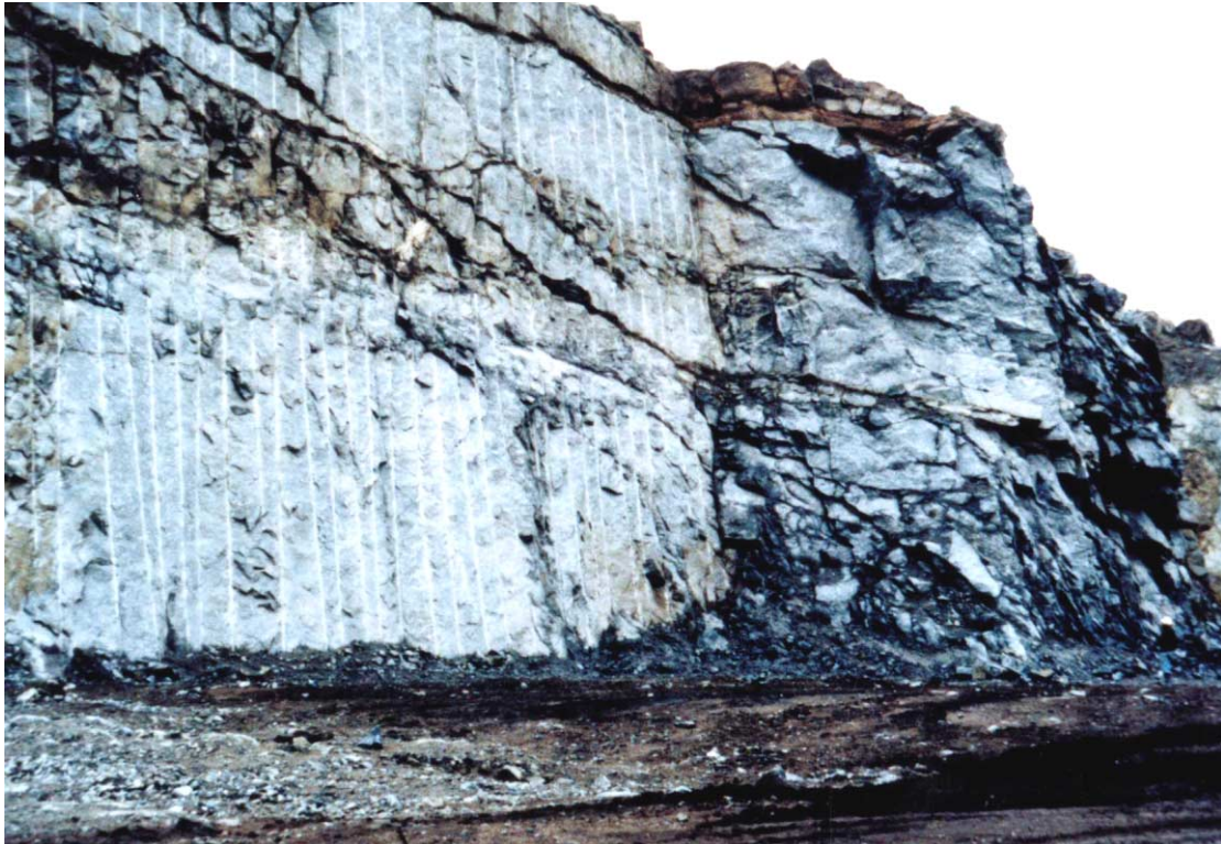
Figure 11.6: Comparison between the results achieved using controlled blasting (on the left) and normal bulk blasting for a surface excavation in gneiss.
