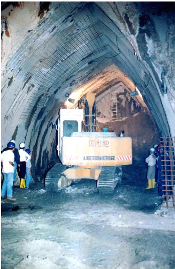
Figure 11.25: Twin side drift and central pillar excavation method. Temporary support consists of double wire mesh reinforced 250 - 300 mm thick shotcrete shells with embedded lattice girders or HEB 160 steel sets at 0.75 - 1 m spacing.
