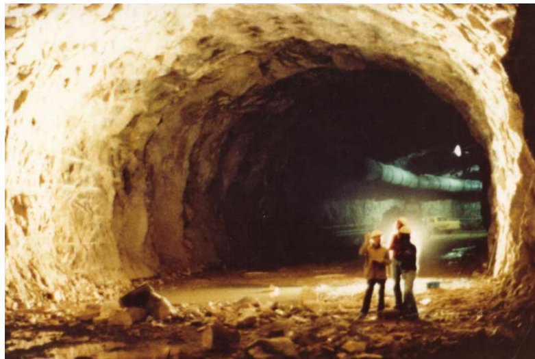
Figure 11.21: Top heading of the 12 m span, 18 m high tailrace tunnel for the Rio Grande Pumped Storage Project.
