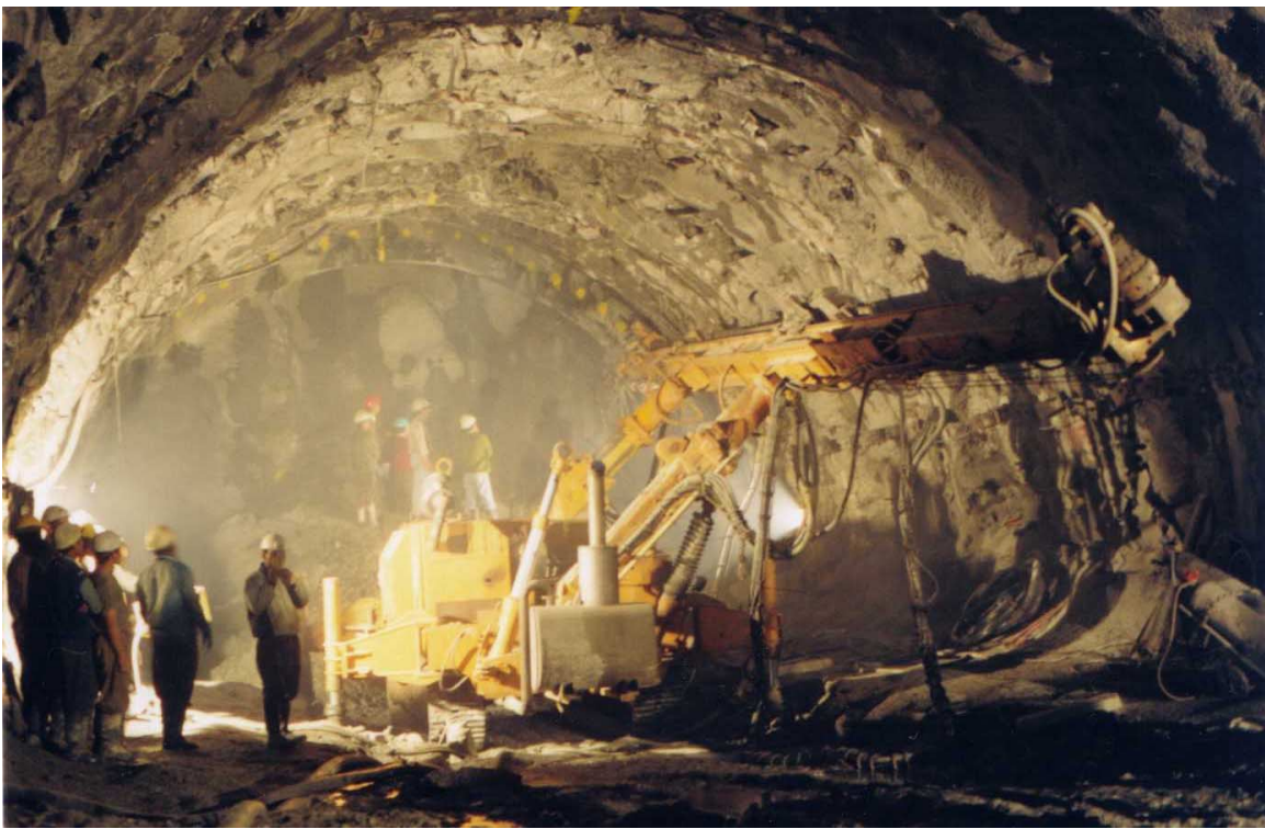
Figure 12.20: Installation of 12 m long 75 mm diameter pipe forepoles in an 11 m span tunnel top heading in a fault zone.
