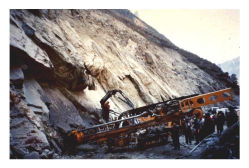
Figure 14.16: Drilling machine for the installation of 40 m long reinforcing cables in 150 mm diameter holes in a dam excavation.
