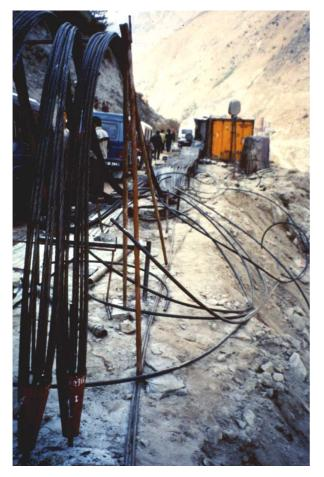
Figure 14.17: 40 m long multi-strand cables with a capacity of 200 tons each being prepared for installation in a dam excavation.
