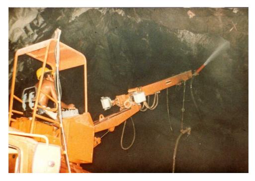
Figure 15.9: A truck mounted shotcrete robot being used in a large civil engineering tunnel. Note that the distance between the nozzle and the rock surface is approximately one metre.
