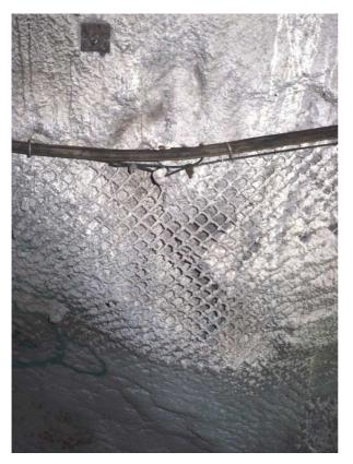
Figure 15.7: Chainlink mesh, while very strong and flexible, is not ideal for shotcrete application because it is difficult for the shotcrete to penetrate the mesh.
