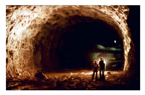
Figure 6.1: The 12 m span 8 m high top heading for the tailrace tunnel was constructed by full-face drill-and-blast and, because of the excellent quality of the massive gneiss, was largely unsupported.
