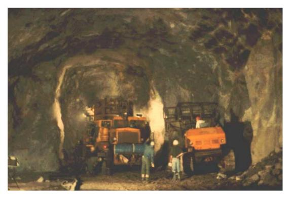
Figure 6.4: A 6 m wide heading driven ahead of the tunnel face to permit pre-reinforcement of potentially unstable wedges in the roof. The seven-boom jumbo is seen working in the heading.
