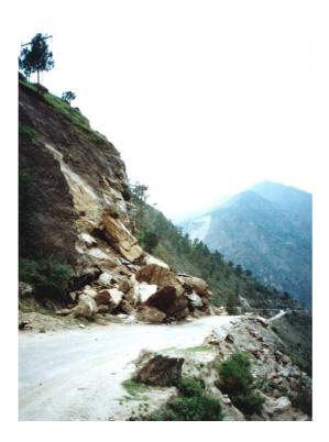
Figure 7.3: A rock slide on a road caused by the undercutting of sheet joints in a granite slope. In hard rocks such as granite, failure can occur very suddenly if the factor of safety of the slope is close to 1. A rise in groundwater levels during a heavy storm or ice jacking in winter may be sufficient to induce failure.
