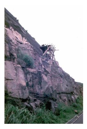
Figure 7.11: Drilling vertical diamond core holes into the Sau Mau Ping slope. These holes were used for geotechnical investigation purposes and also for the installation of piezometers in the rock mass.
