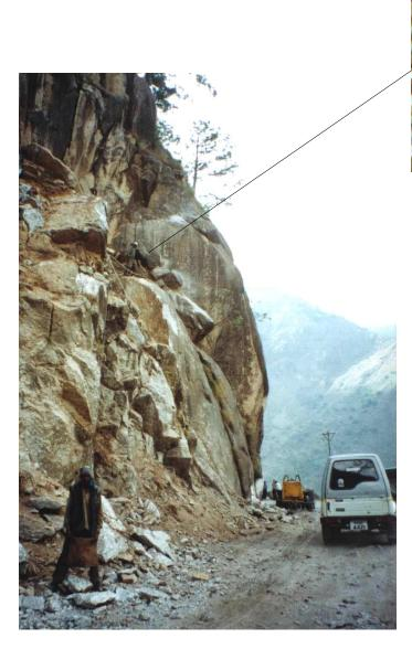
Figure 9.2: Construction on a active roadway, sometimes necessary when there is absolutely no alternative access, increases the rockfall hazard many times over that for slopes without construction or for situations in which the road can be closed during construction.
