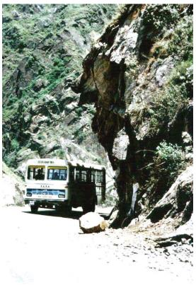
Figure 9.1: A rock slope on a mountain highway. Rockfalls are a major hazard on such highways.
