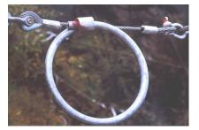
Figure 9.5: Details of a rockfall net system manufactured by Geobrugg of Switzerland.
