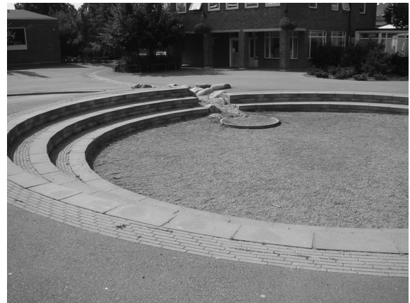
Fig. 2. Structural BMPs in Augustenborg: a) wet pond located between block of flats, b) dry retention basin located at quadrangle (Photos: M. Mrowiec).
