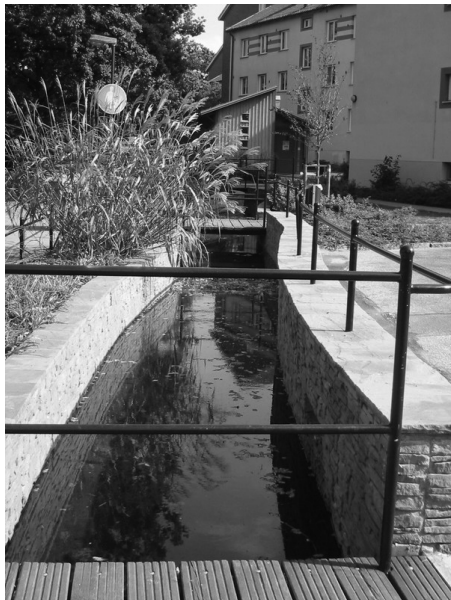
Fig. 3. Open channel system in Augustenborg. (Photos: M. Mrowiec).
