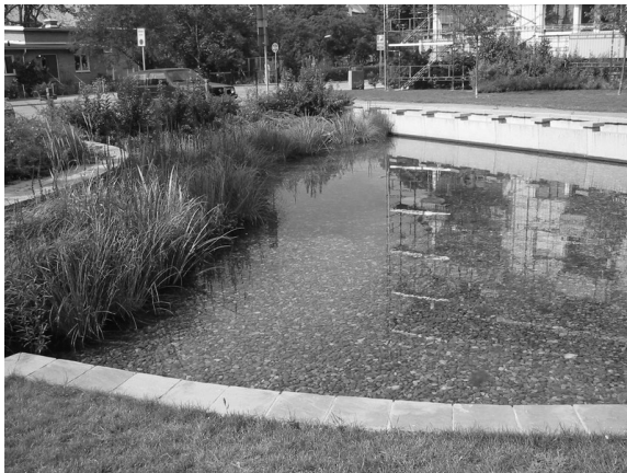
Fig. 2. Structural BMPs in Augustenborg: a) wet pond located between block of flats, b) dry retention basin located at quadrangle (Photos: M. Mrowiec).
