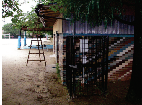
Photo 4. Connection of infiltration facility and cullis water pipe (facility-2).
