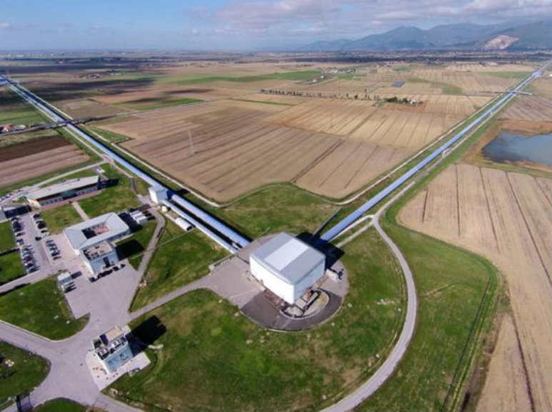
The 1.9-mile-long (3km) arms of the Virgo interferometer nestle in the countryside near Pisa, Italy. The instrument came online August 1 and will help scientists locate future gravitational wave sources. THE VIRGO COLLABORATION
