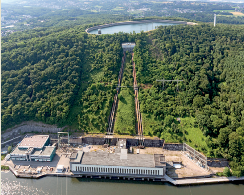
In pumped-storage hydropower stations, water is released to create energy when demand is high.
