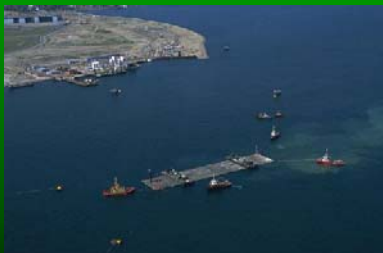
Transport segmentu tunelu
