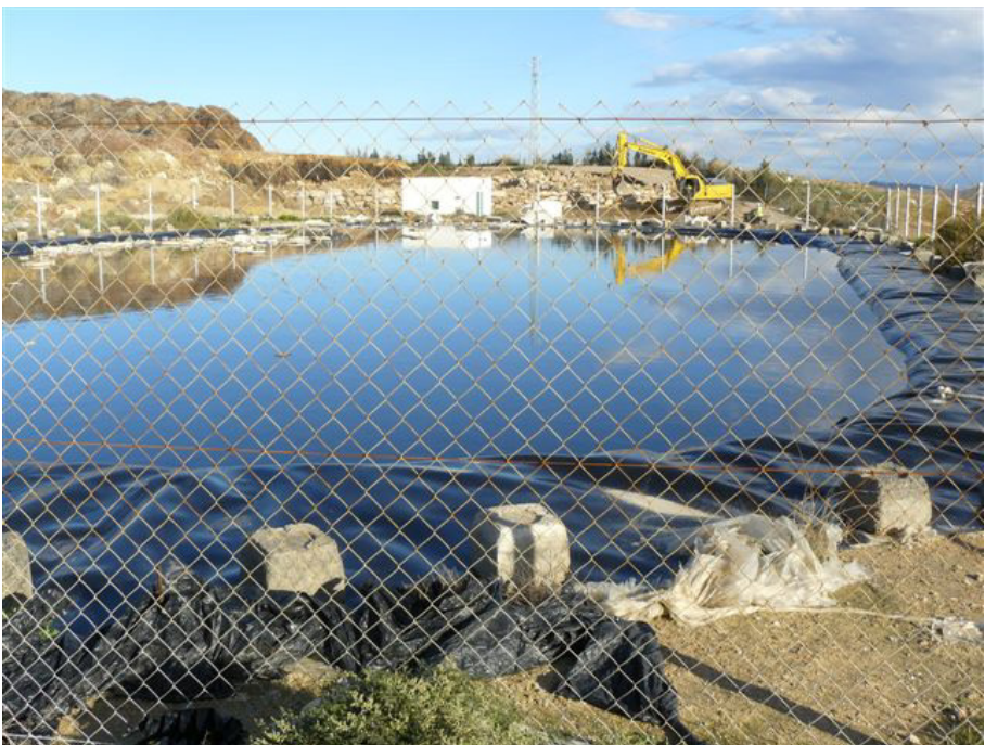
Photos 1 and 2. Aspect of the accumulated plant wastes, showing the leachate emerging in the foreground (a) and a lined leachate pond (b).
