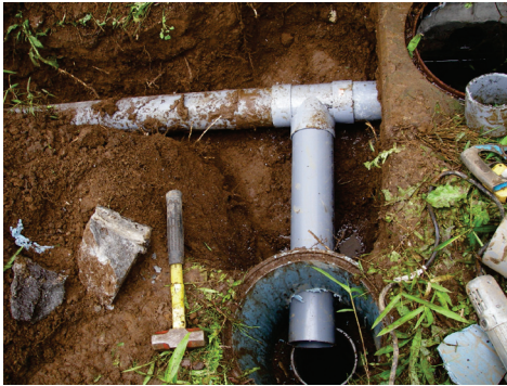
Photo 3. Connection of infiltration facility and cullis water pipe (facility-1).
