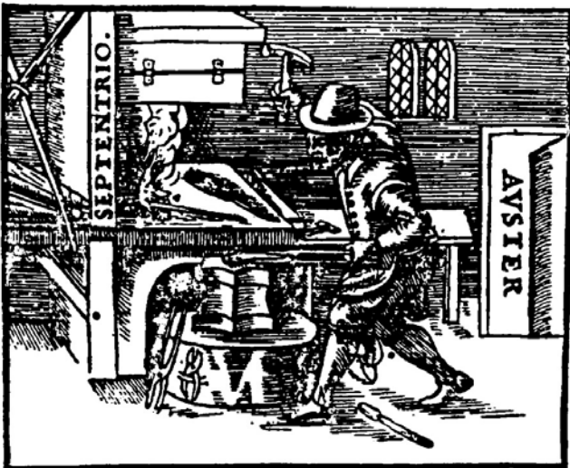
Figure 5 — Method of forging in the earth's magnetic field to produce permanent magnets
