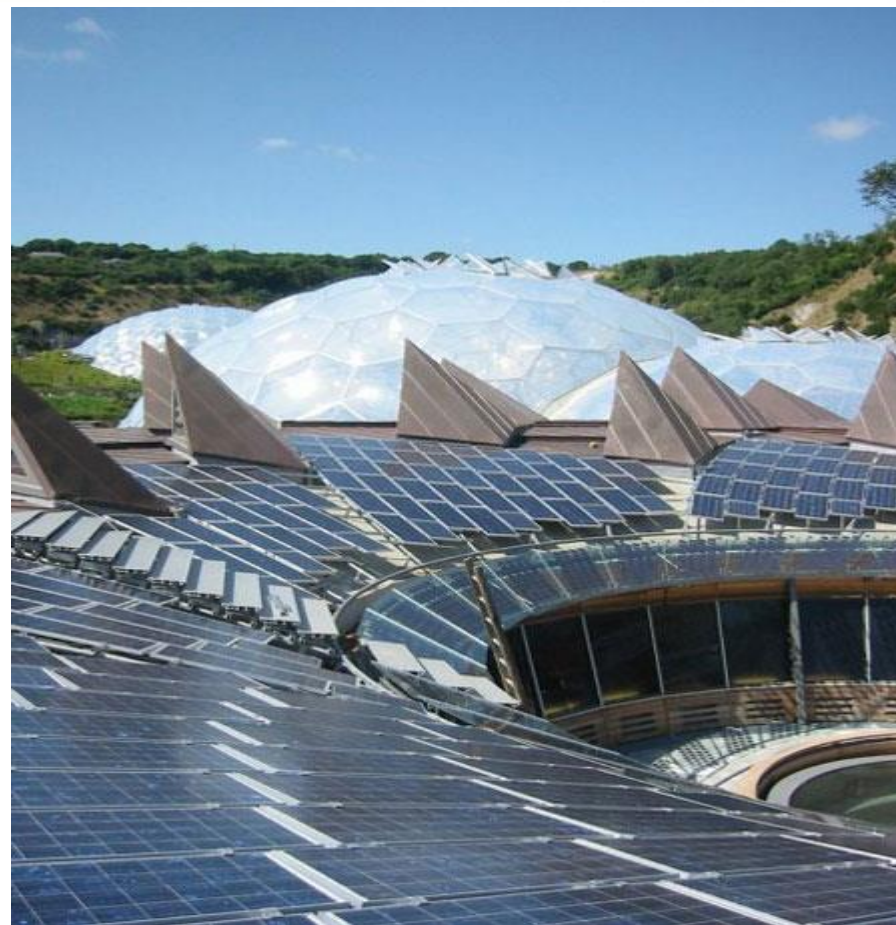
Eden Project, Cornwall, UK http://www.sharpmanufacturing.co.uk
