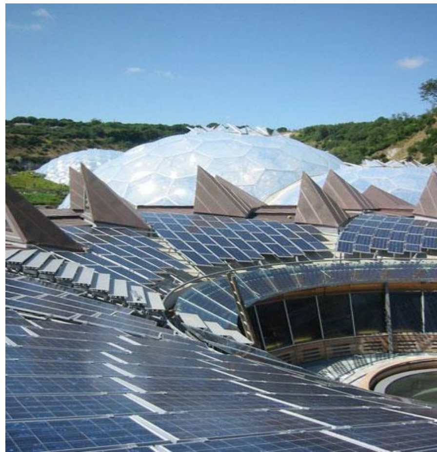
Eden Project, Cornwall, UK http://www.sharpmanufacturing.co.uk
