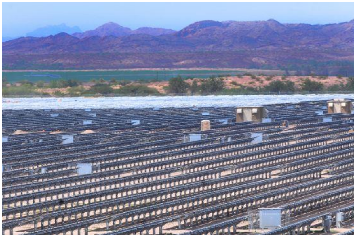
Yuma County, Arizona USA Agua Caliente Solar Project 247MWp (397MWp)
